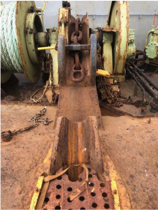
Candidate photo for Deficiency Photo of the Year (Ship type: General cargo/multi-purpose ship; Date: 18/09/2020; Port: Busan)
